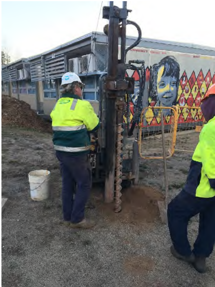
Photo 3: Drilling of borehole 7, looking towards north-west.
