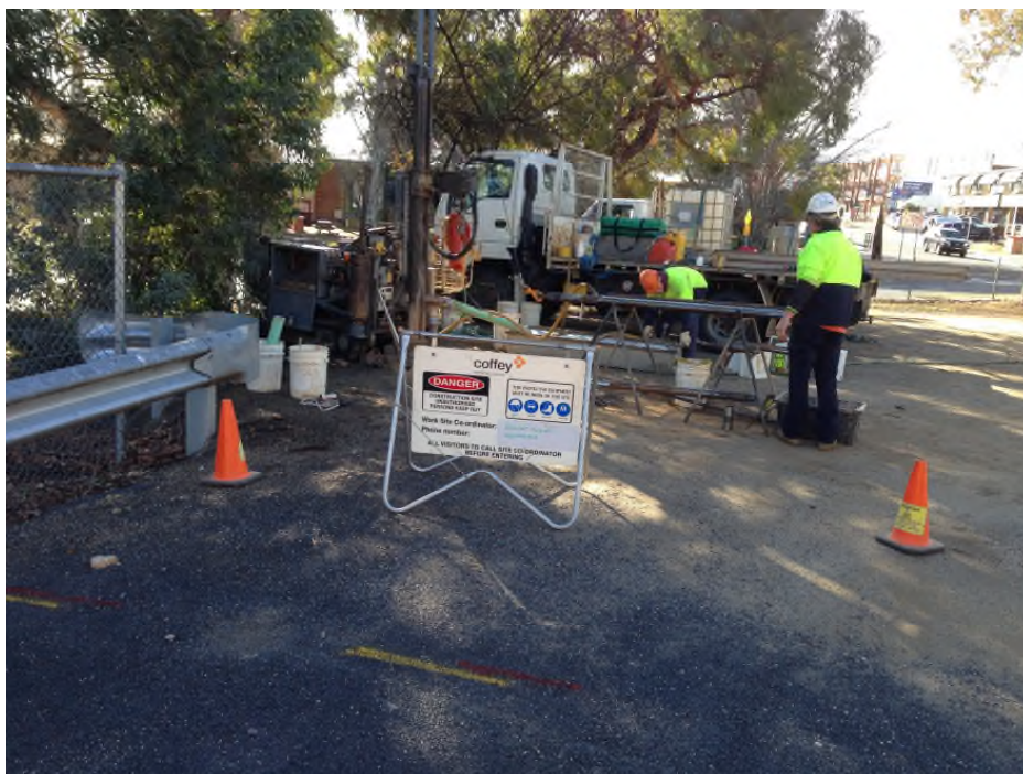
Photo 4: drilling of borehole 4, looking north west
